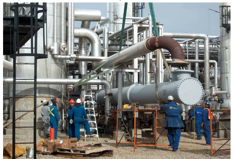
Replacing an Exchanger at the Carstairs Gas Plant
